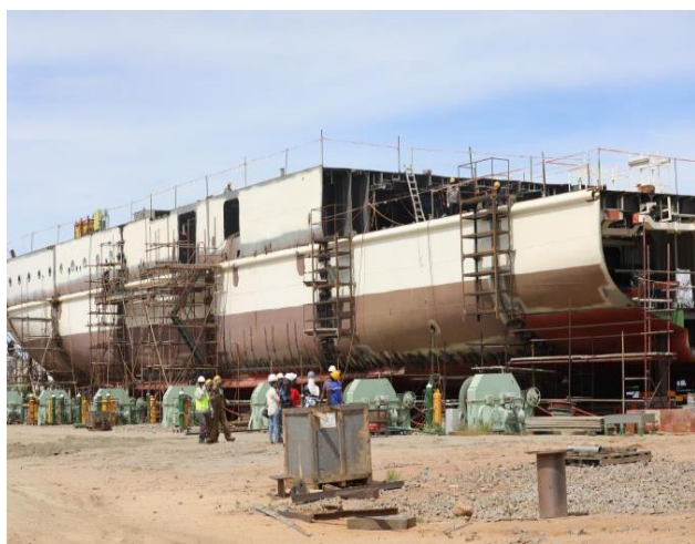
Construction of a new marine vessel (Mv. Mwanza Hapa Kazi Tu)
